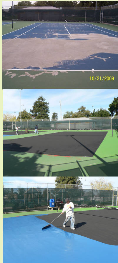
Crack Repair on the Edgewater Courts
